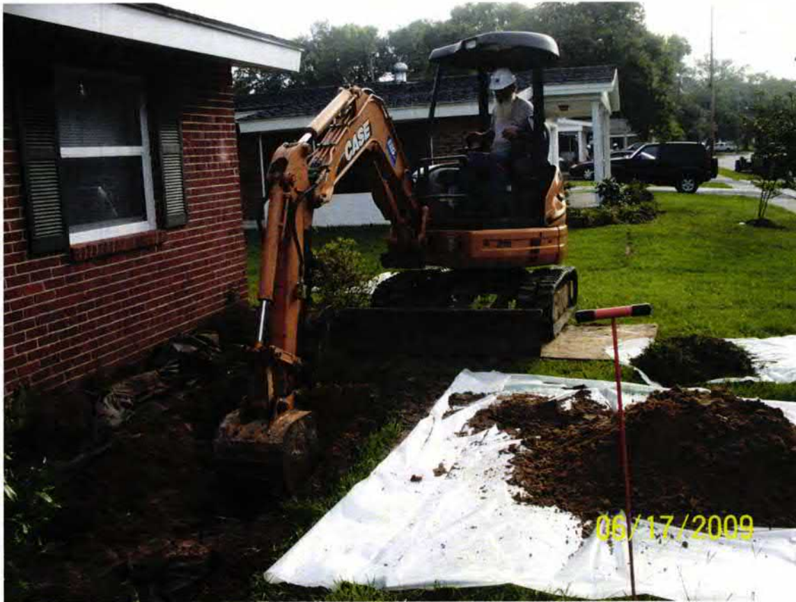
Picture 1: Location of USTs 1111Iris-1 and -2 before removal.
