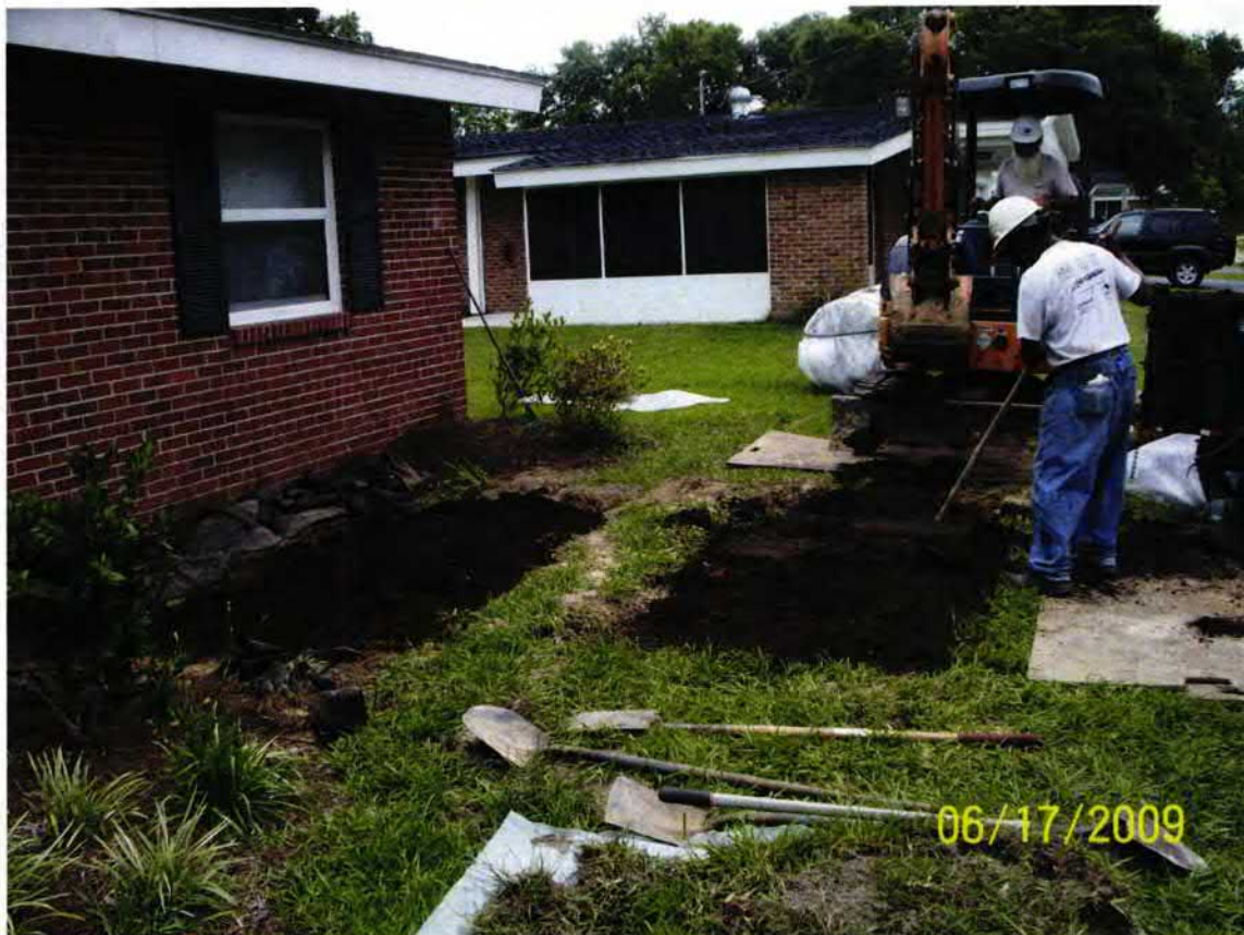
Picture2:UST's 1111 Iris-1 & 2 after removal and during site restoration.
